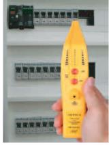
The Circuit breaker which supply the Transmitter circuitry is the one, which, when pointed out by the tip, has the most LEDs lit on the bar-graph and the fastest buzz.
